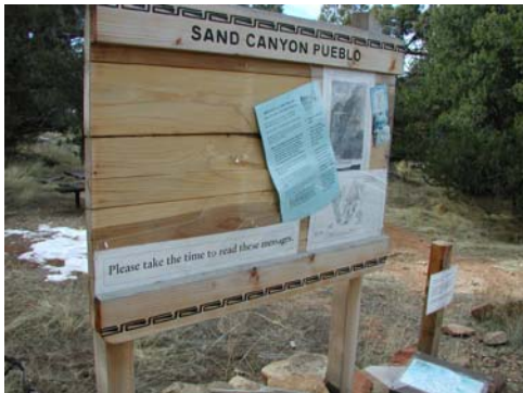
Damaged Sign Board (photo: Kumli)
